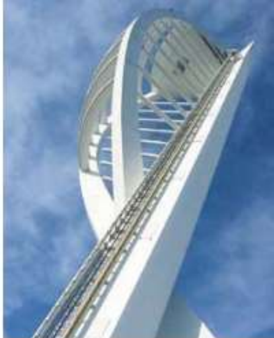
Spinnaker Tower Portsmouth
